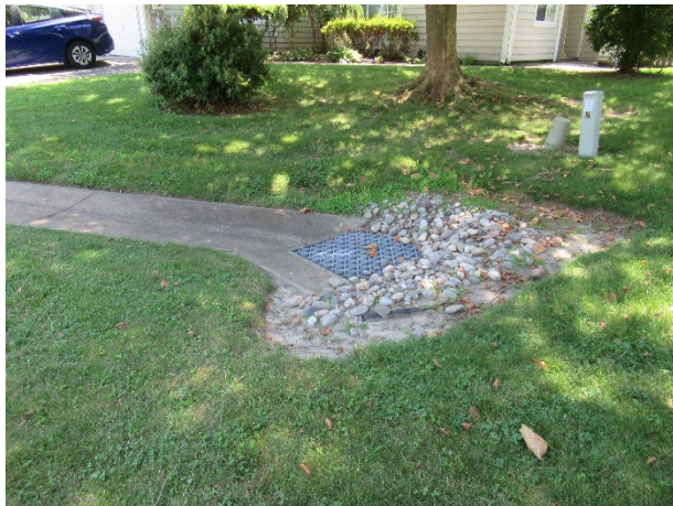
Concrete swale and catch basin
