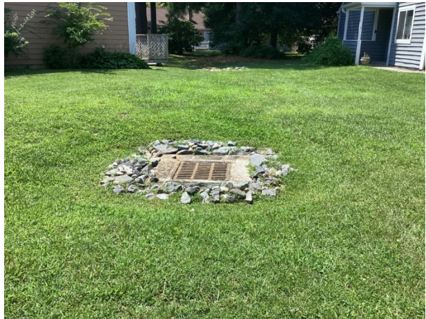
Landscape catch basin
