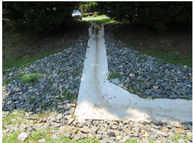
Concrete swale
